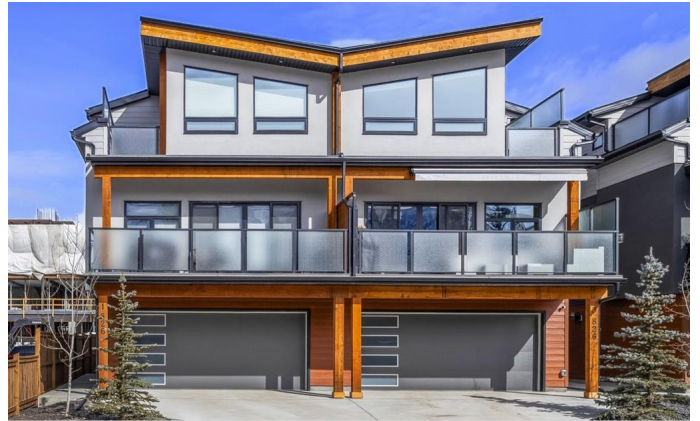
UNIT 1 AT 826 7TH STREET IN CANMORE ALBERTA
